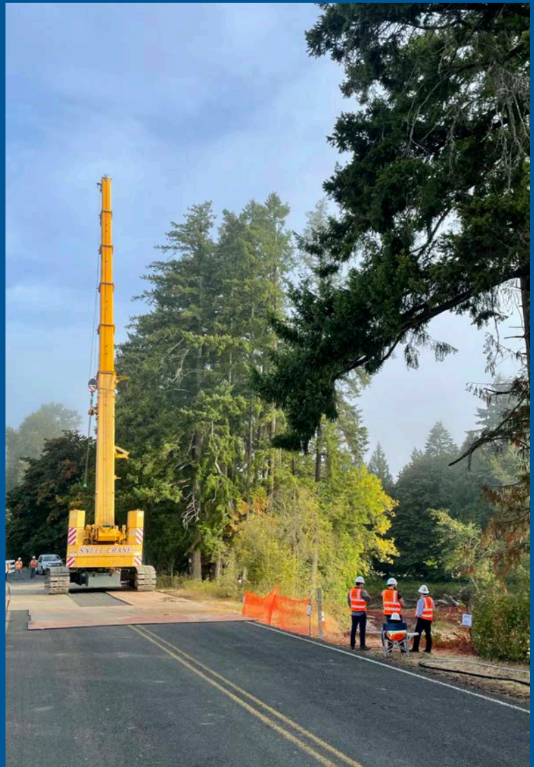
Crane staging during construction.
