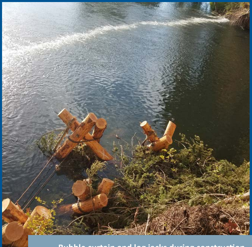
Bubble curtain and log jacks during construction.
