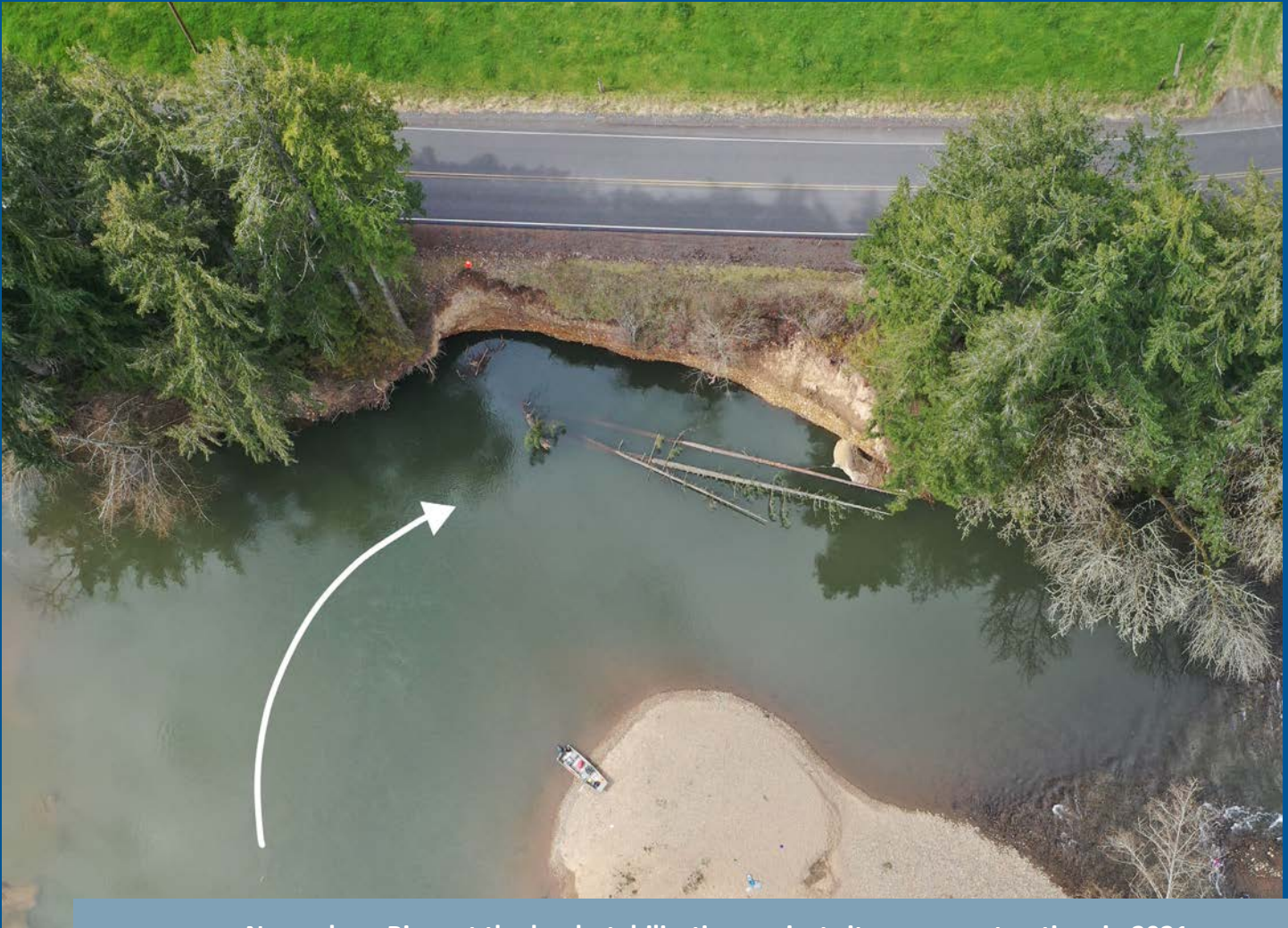
Newaukum River at the bank stabilization project site, pre-construction, in 2021.
