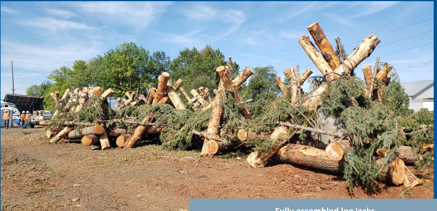
Fully assembled log jacks.
