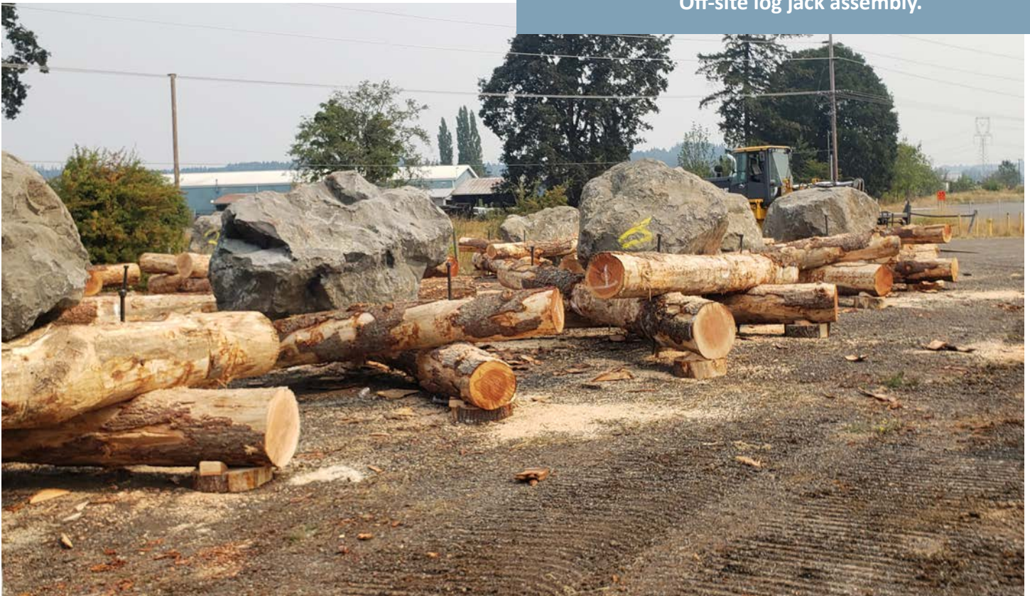
Off-site log jack assembly.
