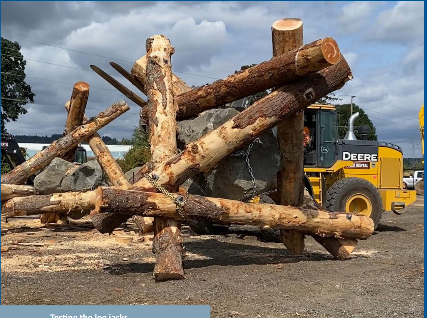
Testing the log jacks.
